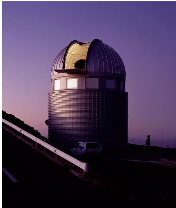
Figure 3.8: Photo showing the 1.2m *Euler* Telescope, at La Silla, Chile. The échelle spectrograph CORALIE is connected at the Nasmyth focus via optical fibre. An imager is located at the secondary focus. Photo courtesy [www.eso.org](http://www.eso.org).
